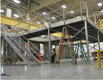
Structural steel, platforms and stairs
